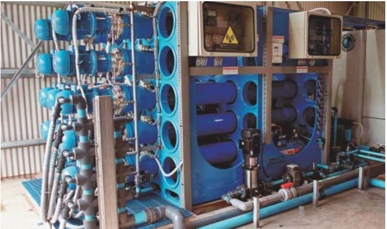
figure 55 - Fresh water made from sea water. The South Australian Water desalination plant at Penneshaw, Kangaroo Island (News Ltd)
