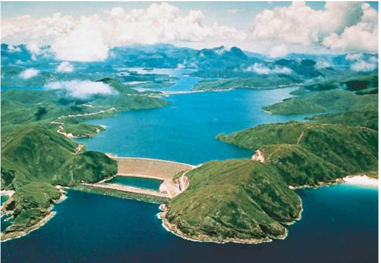
figure 53 - High Island Water Scheme (Courtesy of Hong Kong Government)
