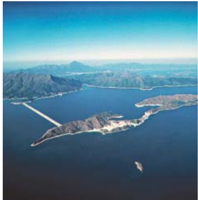
figure 52 - Plover Dam in Hong Kong (Courtesy of Hong Kong Government)
